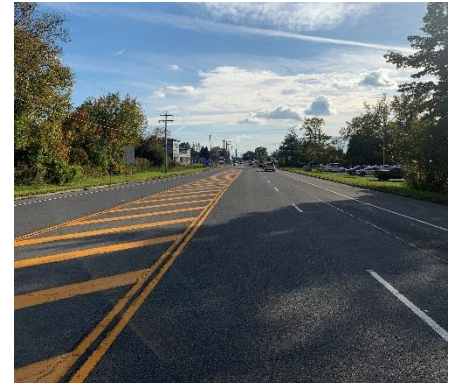
Figure 3.3 US Route 4 Roadway Photo
