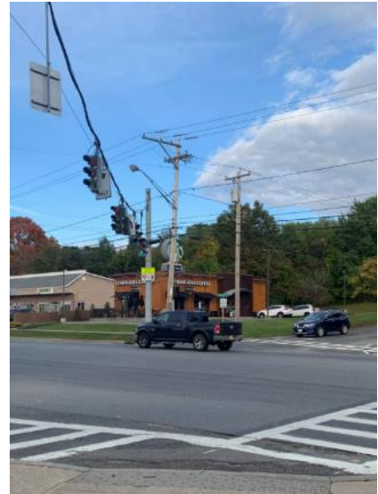
Figure 6.2 US Route 4 Traffic Signal at Grandview Drive
